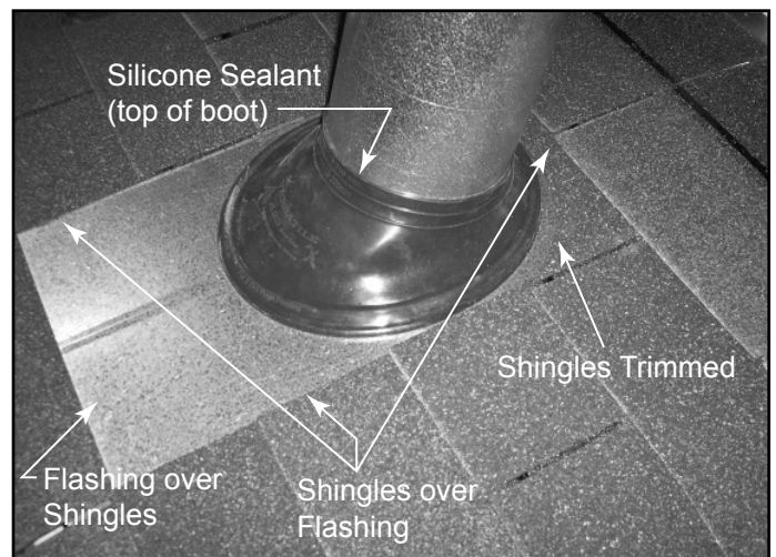
Figure 10.22 Installation Complete
